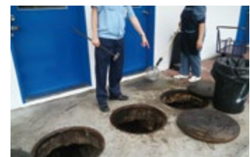
Checking a cafeteria grease trap
