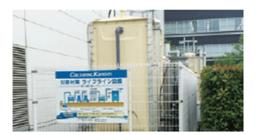
Groundwater membrane filtration system installed at R&D Center and Headquarters
